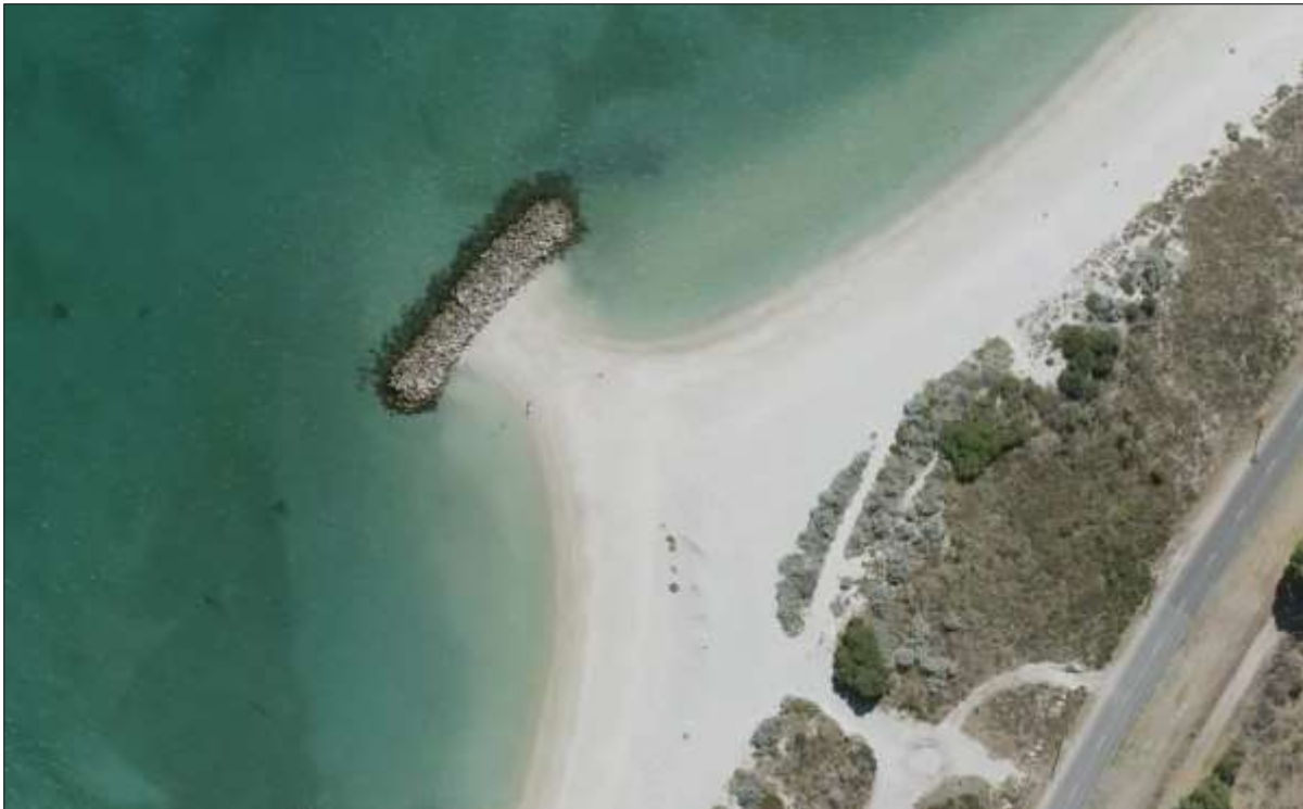
Figure 4-4 Offshore breakwater at Kwinana Beach, WA
