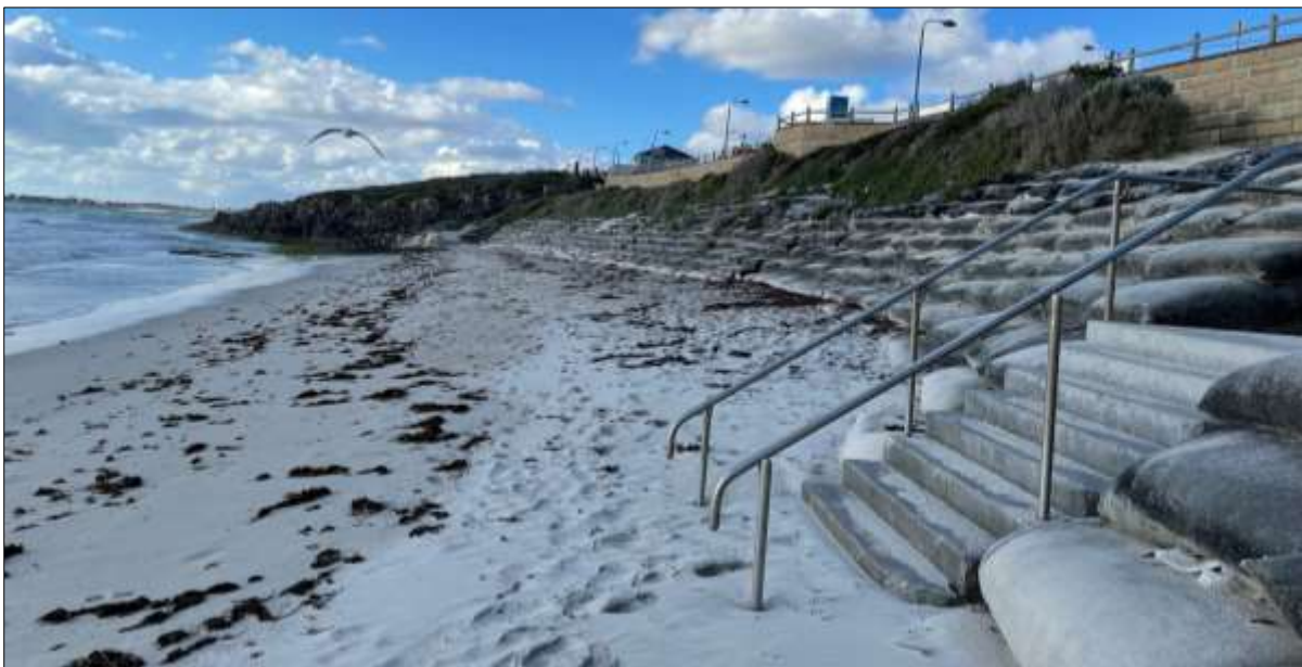
Figure 4-5 GSC seawall at Watermans Bay Beach
