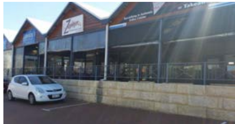
Articulation of coastal form within southern section of Flora Terrace
