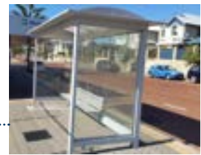
Existing bus shelter north within pedestrian pathway
