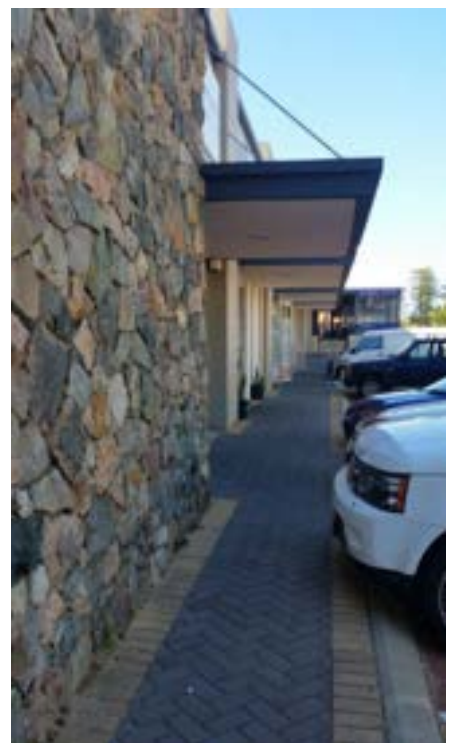
Awning structures south of Castle St
