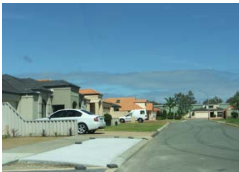
Plate 4 Stirling (St Anthony's Estate), R40 – single storey developments with parapet (common) walls.
