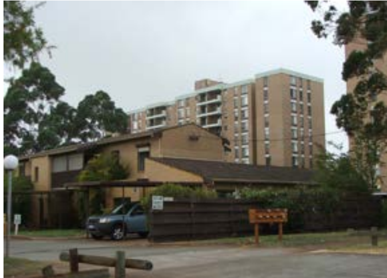
Plate 8 : Glendalough R60 — multiple dwellings in foreground; high rise in background (assessed under previous, high density coding)
