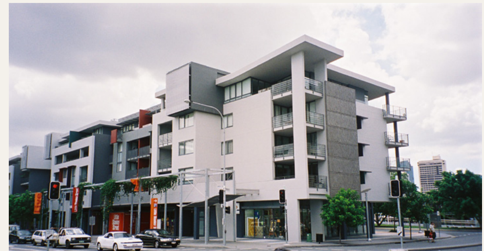
Examples of roof forms that integrate with the overall building design and assist in reducing building mass
