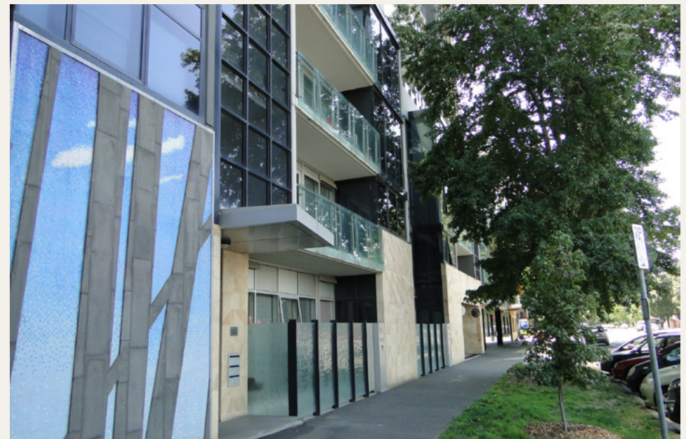
Buildings providing adaptable ground floor to allow for change of use over time
