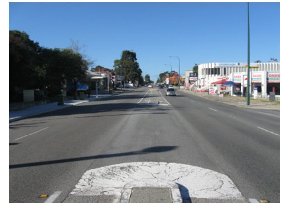
Poor public realm amenity and streetscape, unfriendly pedestrian environment and lack of street trees and soft landscaping. Big box scale and built form of development not of human scale.
